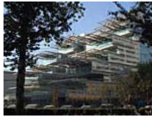
MARIO CUCINELLA ARCHITECTS, CINA I SIEEB SINO ITALIAN ECOLOGICAL AND ENERGY EFFICIENT BUILDING
