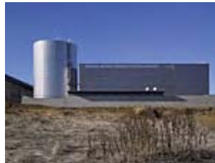
SKIDMORE&OWINGS&MERRILL, USA UNIVERSITY OF CALIFORNIA, MERCED, CENTRAL PLANT
