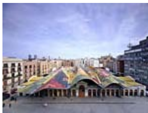
MIRALLES TAGLIABNE, SPAGNA REHABILITATION OF SANTA CATERINA MARKET
