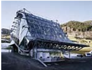
DRIENDL ARCHITECTS, AUSTRIA GALZIGBAHN CABLE CAR STATION
