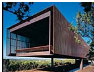
SEAN GODSELL ARCHITECTS, AUSTRALIA SIR ANDREWS BEACH HOUSE
